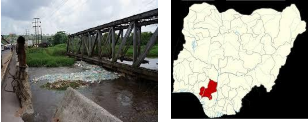
Map 1. Ikpoba River in Benin City. Industrial effluent (brewery waste) discharged into the river.
